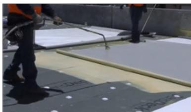
Spray application requires airless spray equipment. Roller application is also acceptable.
