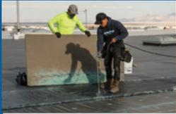
**CAV-GRIP® III Introduced for EPDM:** This VOC-compliant and very low-odor primer/adhesive represented a big leap forward in jobsite productivity.
