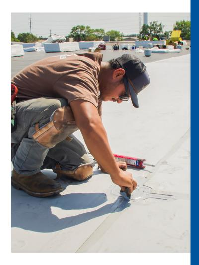
a very fast flash-off time and considerable labor savings when compared to traditional bonding adhesive. Paul's chose to use the smaller #40 cylinders for easy portability on the roof.
