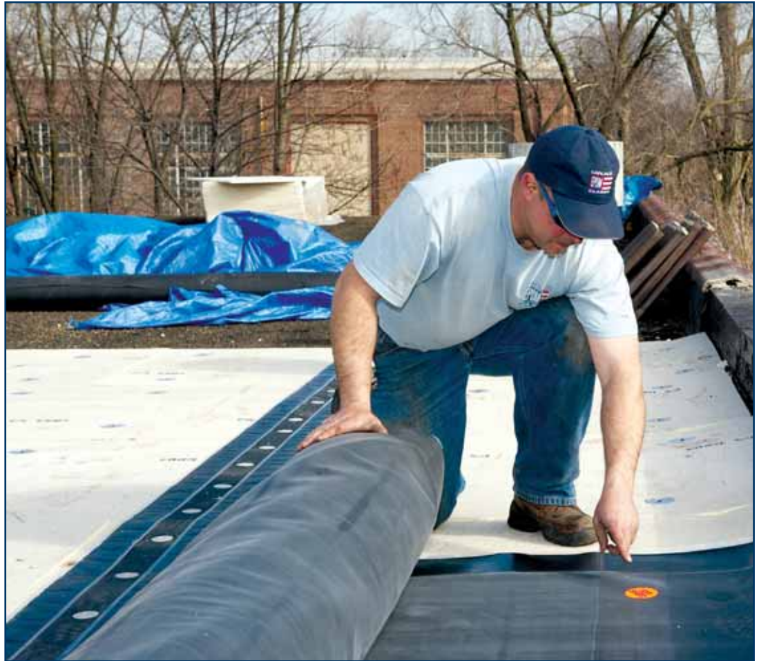
Cover an existing built-up roof and add thermal value by applying additional insulation under the EPDM membrane. The sheeting shown has factory-applied (seam) tape for faster installation with greater peel and shear strength.
