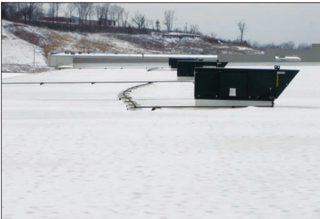
This warehouse in St. Louis, Mo., had significant snow and ice pack movement, dislodging gas lines running across a white roof.
