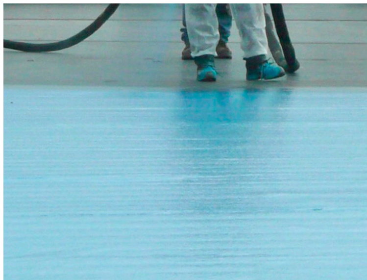
Fig 1. Full Spray Application
