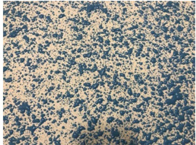
FIG 1. CORRECT COVERAGE – SPLATTER APPLICATION
