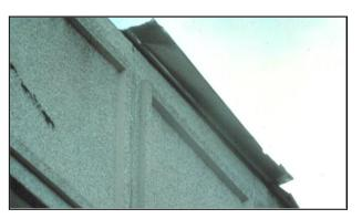
Another key finding from the study included discovery of cleat gauges that were less than those recommended by FM Global 1-49 and ANSI/SPRI ES-1. The committee also found that 95 percent of roof failures were caused by poor workmanship and substituted materials.
