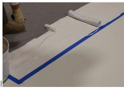
INSTALL BOTH LAYERS OF PRE-CUT LIQUISEAL Flashing Fleece, EMBEDDED IN RESIN (SEE <u>LF-13.2A</u>).
