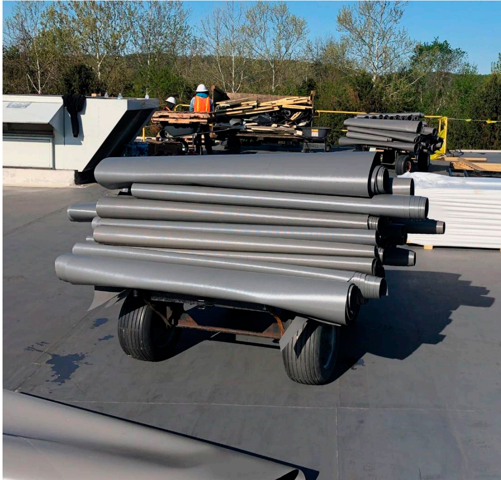
Membrane is prepared and palletized, secured and loaded on a trailer.
