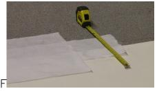
CUT TWO PIECES OF LIQUISEAL Flashing Fleece, (FOR DIMENSIONS SEE LF-13.2A).
