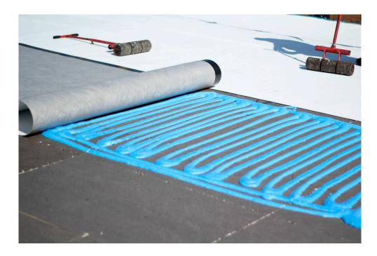
3. Allow the adhesive to rise up approximately 1/4" to 3/4", depending on dispensing method, and develop string-time prior to setting insulation boards into adhesive.
