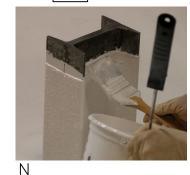
TOUCH UP AS NEEDED TO ENSURE ENTIRE FLEECE IS COMPLETELY SATURATED.
