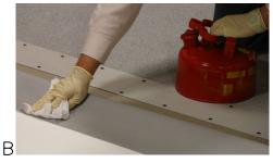
PROPERLY CLEAN WITH MEMBRANE CLEANER PRIOR TO WELDING.
