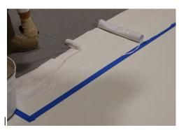
INSTALL BOTH LAYERS OF PRE-CUT LIQUISEAL Flashing Fleece, EMBEDDED IN RESIN (SEE LF-13.2A).
