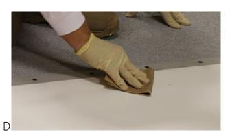
USE SAND PAPER GRIT # 60 TO ABRADE THE AREAS TO WHICH THE LIQUISEAL LIQUID FLASHING RESIN WILL BE APPLIED.
