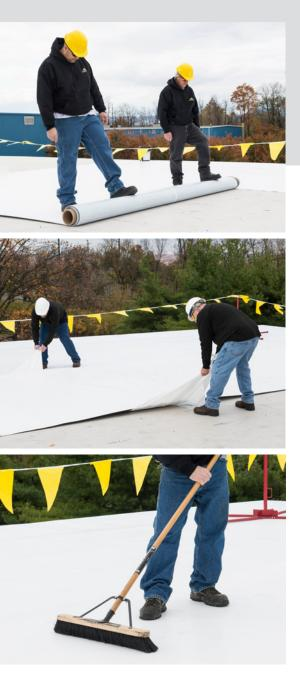
Versico's VersiWeld® QA TPO roofing membrane with pre-applied adhesive combines the energy efficiency and durability you expect from Versico's VersiWeld TPO with the easiest installation in the industry. Our quick-applied technology saves labor and improves membrane performance, which translates into satisfied building owners.
