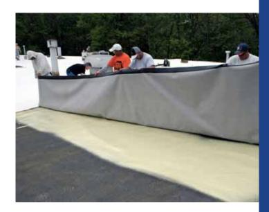
of waterproofing insulation which also acts as an air barrier and eliminates thermal bridging. Carlisle SynTec Systems' FAST Adhesive was applied to the SPF, after which the FleeceBACK membrane was set and rolled into the adhesive.
