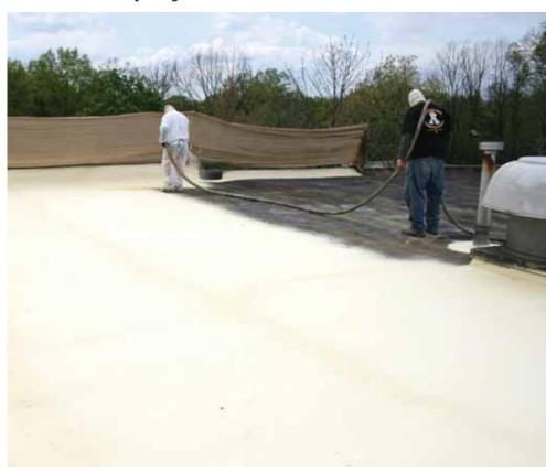
Spray Polyurethane Foam (SPF) roofing systems have been around since the 1960's, and for good reason. Roofing professionals generally agree that the most significant benefits of SPF are its watertight performance, resistance to leaks, and insulation properties. SPF also offers high compressive strength, is lightweight, self-flashing, durable and long-lasting. All these features have made it a very popular roof system over the past several decades.
