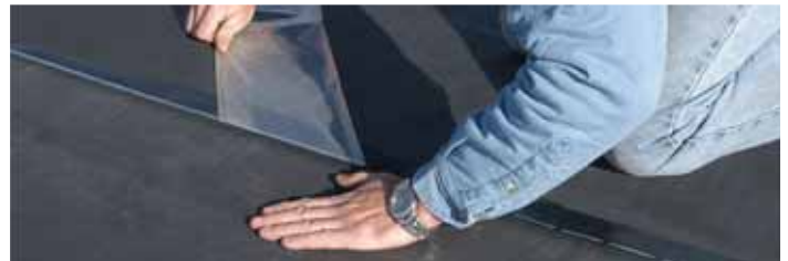
Seams completed with Factory-Applied Tape go together smoothly, resulting in fewer wrinkles.
