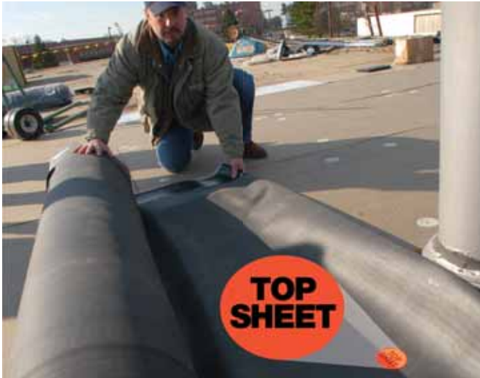
Locate the orange "TOP SHEET" sticker on 2-packs to ensure proper roll-out.
