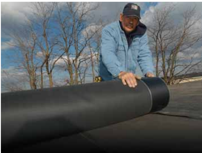
Seam set-up is simple using pre-marked sheets with Factory-Applied Tape.
