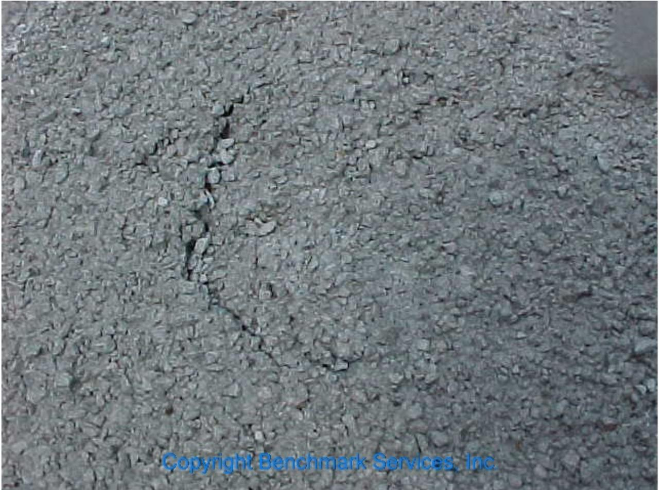
**Figure 3 - Hail Damaged granule surfaced SPUF Roof**
