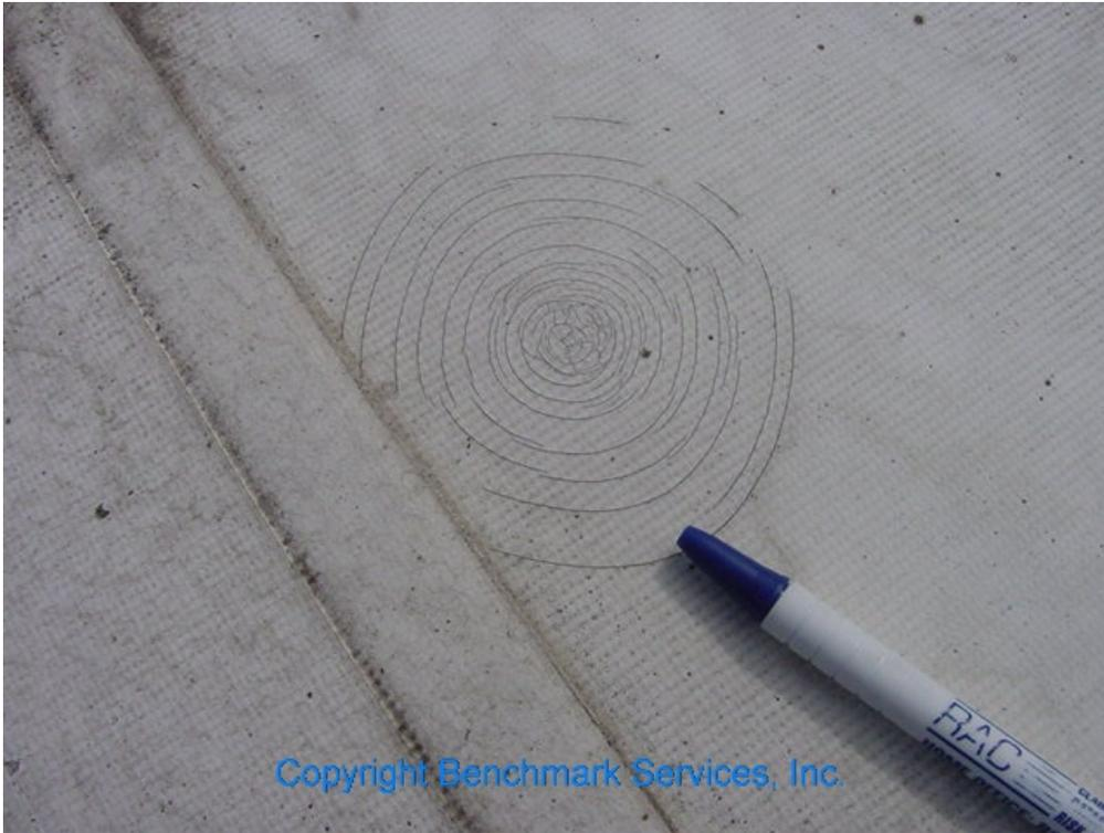
**Figure 6 - Reinforced PVC Membrane Hail Fractured**
