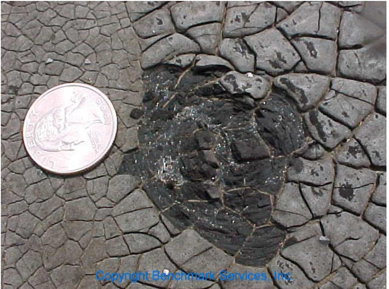
**Figure 2 - Built -up roof damaged by 1 1/2" hail**
