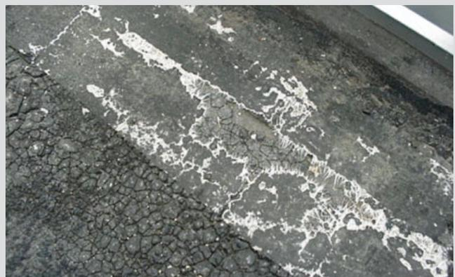
Ponding Water Extracts Oils from Asphalt
