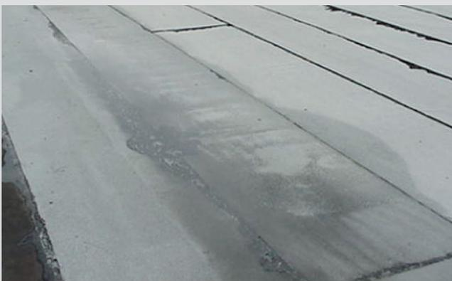
Ponding Water Accelerates Granule Loss
