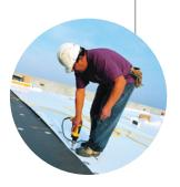
EPDM with Factory-Applied Tape (FAT™) was developed, improving seaming productivity by approximately 75%.
