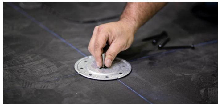
**Step 2:** Install the U-Anchor Plate with the type and number of fasteners specified by your design professional, securing the plate to the roof deck through the existing roofing system.
