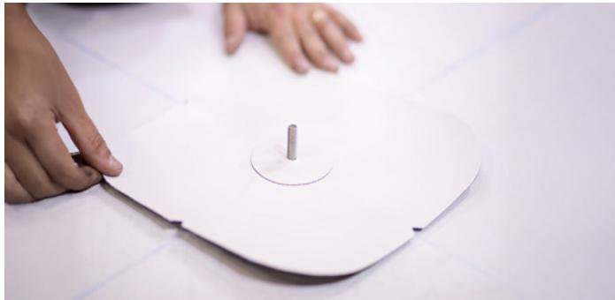
**Step 2:** Fold the flashing membrane up to expose the U-Anchor plate. Install the U-Anchor Plate with the type and number of fasteners specified by your design professional, securing the plate to the roof deck through the existing roofing system.
