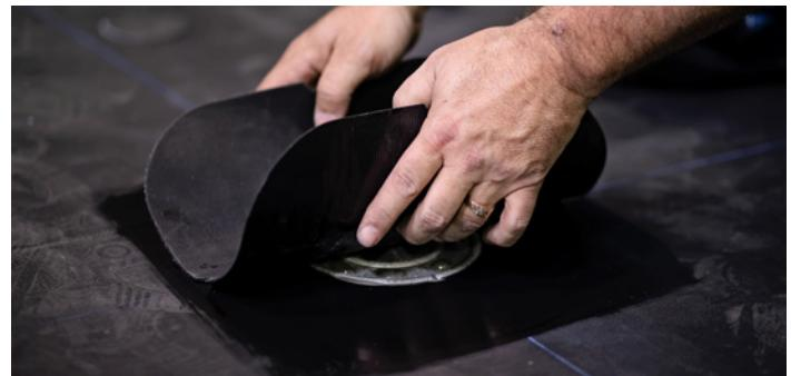
**Step 6:** Remove the release liner by pulling it out at a 90° angle from beneath the flashing, taking care not to shift the material. Press the flashing firmly onto the roof surface and U-Anchor plate, smoothing it with your hands to avoid wrinkles and air pockets.
