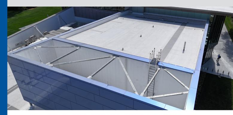
are three sections with concrete decks that house a variety of mechanical equipment, which all had to be carefully flashed. In addition, each required tapered insulation and crickets for drainage around the mechanical curbs.
