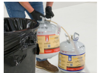
Shaking of A-side and B-side tanks
