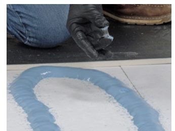
Performing the string-tie test
