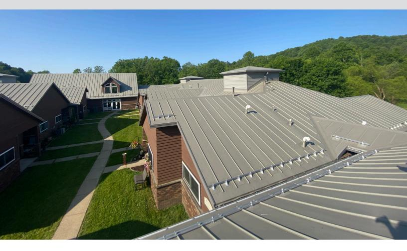
The original specification, developed by Michael Lichy of Lichy & Associates of Cranberry Township, Penn., called for a standing seam metal roof lifted an inch over the existing roof for air circulation, which was one of the critical issues with the previous roofing systems.
