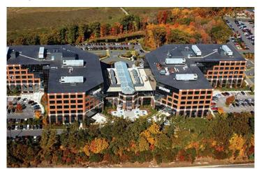
Black EPDM helps to reduce heating costs in northern climates, which are typically 3-5 times greater than air-conditioning costs.
