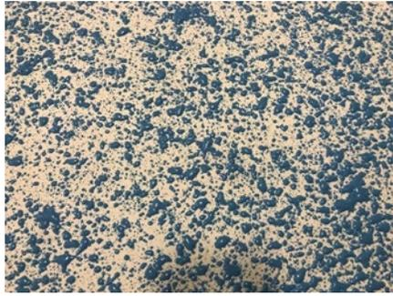
**Fig 3.** Correct Coverage – Splatter Application
