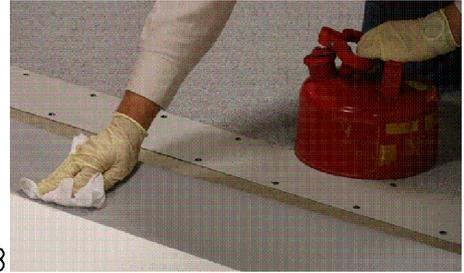
PROPERLY CLEAN WITH MEMBRANE CLEANER PRIOR TO WELDING.
