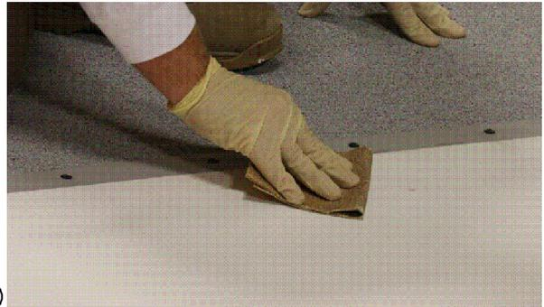
USE SAND PAPER GRIT # 60 TO ABRASE THE AREAS TO WHICH THE LIQUISEAL LIQUID FLASHING RESIN WILL BE APPLIED.
