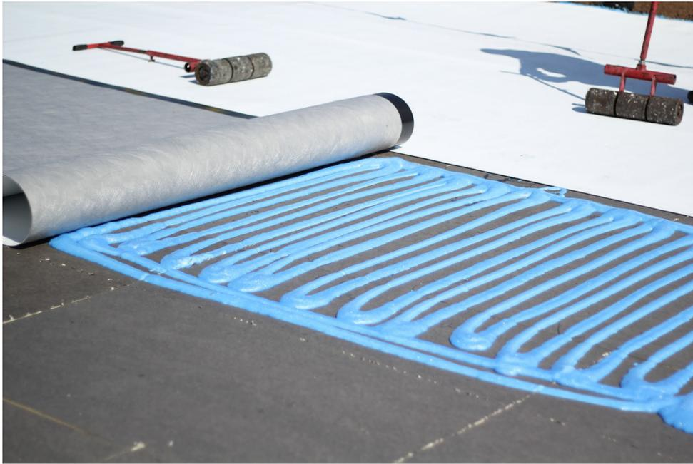
3. Allow the adhesive to rise up approximately 1/4" to 3/4", depending on dispensing method, and develop strings prior to setting insulation boards into adhesive.
