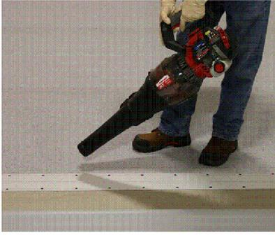
INSTALL COATED SHEET METAL STRIPS WITH THREADED FASTENERS. REFER TO TABLES ON SHEETS [ATTACHEMIN 1-2](#) FOR DETAILED INSPECTION, CLEANING AND PRIMING FOR DIFFERENT MATERIALS WITHIN THE FLASHING AREAS.
