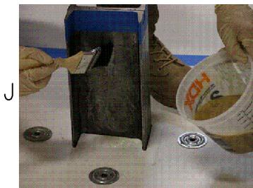
PRIME I-BEAM AND METAL PLATES. ENSURE AMBIENT AIR TEMPERATURE IS 40° & RISING. ALLOW PRIMER TO CURE UNTIL TACK-FREE.
