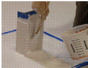
IMMEDIATELY APPLY A 2ND COAT OF LIQUISEAL Liquid Flashing Resin ENSURING THE FLEECE IS COMPLETELY SATURATED.
