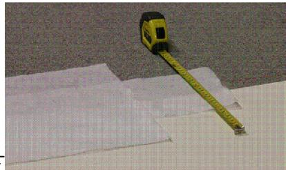
CUT TWO PIECES OF [LIQUISEAL Flashing Fleece](#), (FOR DIMENSIONS SEE [13.2A](#)).
