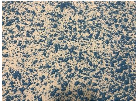
Fig 3. Correct Coverage – Splatter Application
