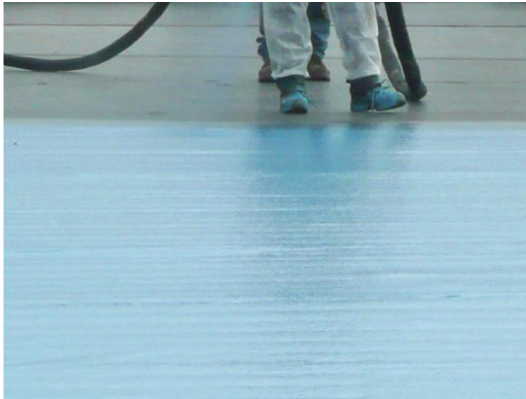
Fig 1. Full Spray Application
