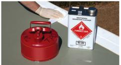
Clean the surface to be painted using Versico's Weathered Membrane Cleaner and allow to dry thoroughly.
