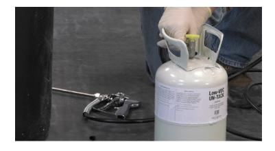
When removing the spray tip of the gun for cleaning or replacement, it is not necessary to relieve the pressure in the gun and hose assembly. Make sure the safety stop on the trigger is positioned to not allow the gun to operate. Wear safety glasses during this procedure and anytime while spraying adhesive.
