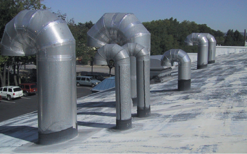
Before: Overview of existing 39-year-old Versico roofing system.
