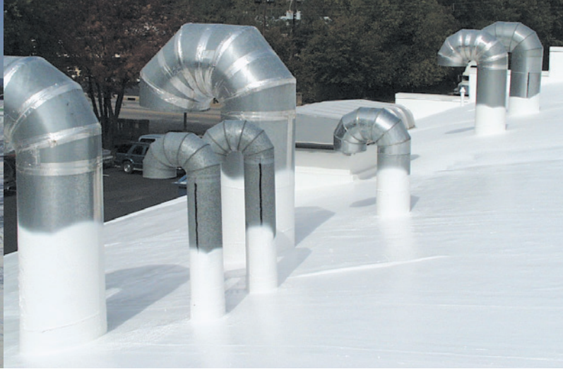
After: Completed restoration.
