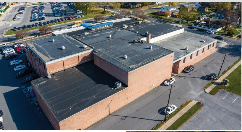
The existing ballasted EPDM inverted roof membrane assembly (IRMA) was at the end of its service life after 37 years. The existing system was installed on a concrete deck and included loose-laid EPDM, four to six inches of extruded polystyrene (XPS) insulation, protection mat, and gravel ballast over the top.
