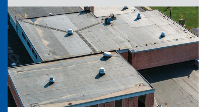
insulation, which was adhered with Flexible FAST Adhesive. In addition, they installed several crickets on the roof for better drainage to the existing rooftop drains.
