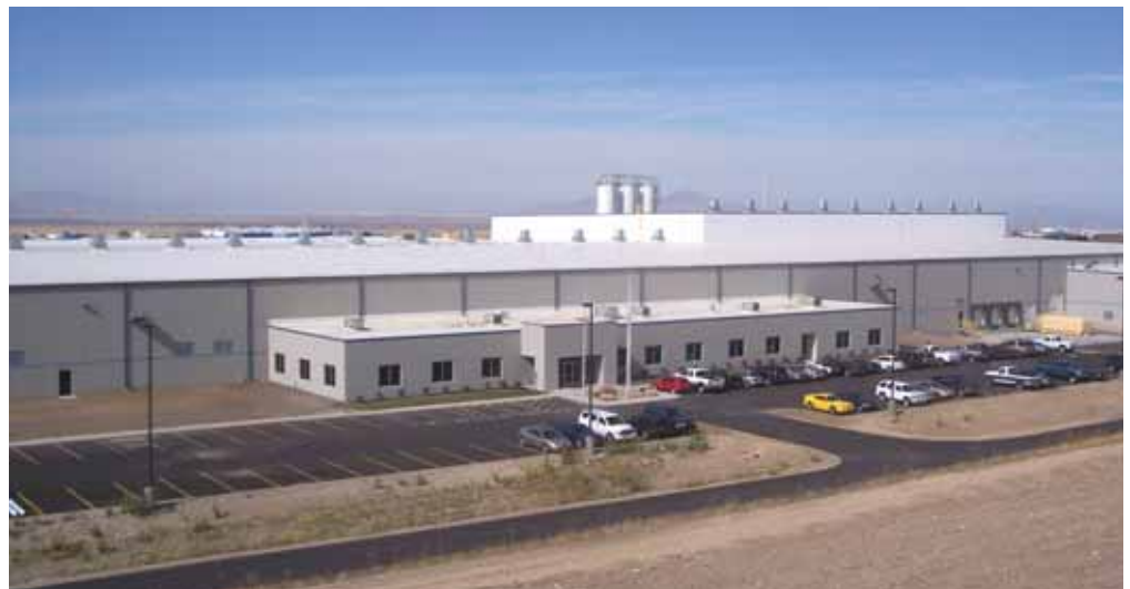
Carlisle SynTec opened a second TPO line at the Tooele, Utah plant in early 2008 to meet the demand for TPO.
