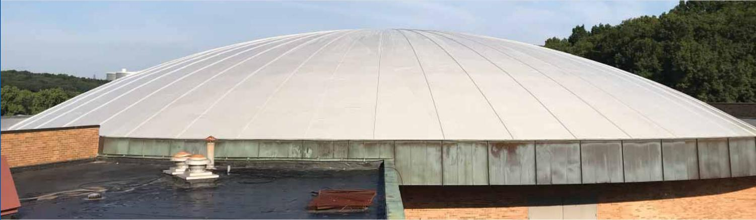
They chose a gray FleeceBACK KEE HP PVC system adhered with Flexible FAST Adhesive because of its long service life, exceptional weatherability, flexibility, and toughness, and excellent resistance to wind uplift, hail, and punctures. PVC Contour Ribs, which simulate the look of a standing seam metal roof, were added to the design to give the dome an “architectural” look and to showcase the unique roof section.
