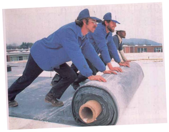
Now contractors have the option of a 90-mil EPDM, which has twice the puncture resistance of the original 45-mil rubber and contains the most weathering material of any single-ply membrane on the market.
