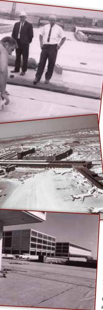
asphalt-based roofs and lowered the quality of available asphalt. EPDM was cost-effective and simple to install, and quickly became known for its exceptional hail resistance, UV stability, and weathering resistance due to the cross-linked nature of its chemistry and the UV-absorbing power of its raw materials.
