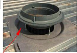
VOID UNDER DRAIN FILLED WITH RIGID BOARD INSULATION AND SET IN CONSTRUCTION ADHESIVE. BUILD SQUARE CURB AROUND THE DRAIN.
