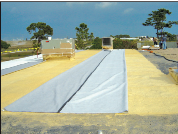
Sure-White™ EPDM FleeceBACK is positioned to allow the application of FAST Adhesive.
