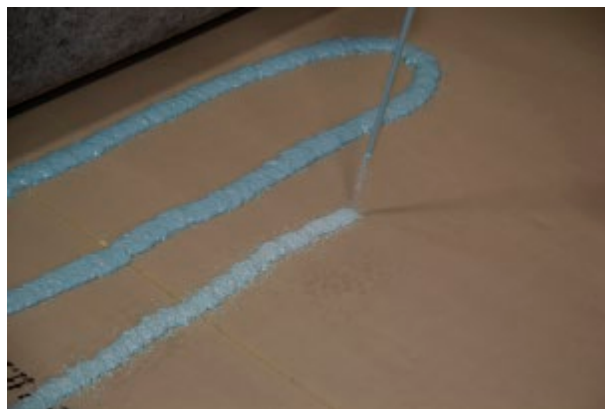
Fig 2. Bead Application
