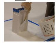
IMMEDIATELY APPLY A 2ND COAT OF LIQUISEAL Liquid Flashing Resin ENSURING THE FLEECE IS COMPLETELY SATURATED.
