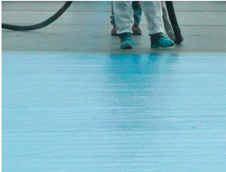
Fig 1. Full Spray Application
