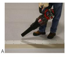
INSTALL COATED SHEET METAL STRIPS WITH THREADED FASTENERS. REFER TO TABLES ON SHEETS ATTACHEMTN 1-2 FOR DETAILED INSPECTION, CLEANING AND PRIMING FOR DIFFERENT MATERIALS WITHIN THE FLASHING AREAS.
