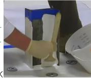
IMMEDIATELY APPLY A 2ND COAT OF LIQUISEAL Liquid Flashing Resin ENSURING THE FLEECE IS COMPLETELY SATURATED.
