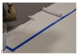
INSTALL BOTH LAYERS OF PRE-CUT LIQUISEAL Flashing Fleece, EMBEDDED IN RESIN (SEE LF-13.2A).
