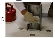
REMOVE ALL GRINDING DUST, CLEAN METAL & MEMBRANE WITH CLEAN RAGS & MEMBRANE CLEANER.
