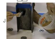
PRIME I-BEAM AND METAL PLATES. ENSURE AMBIENT AIR TEMPERATURE IS 40° & RISING. ALLOW PRIMER TO CURE UNTIL TACK-FREE.
