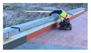
was installed up the wall about a foot and terminated with a termination bar. A coping cap was then installed over the top of the parapet wall sections.
