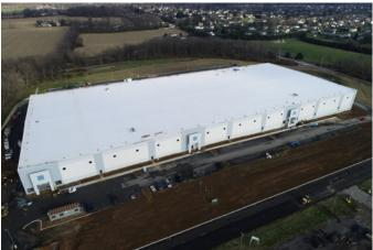
"The 16-foot rolls were better for production, and there were fewer seams to weld. We were able to install iso for three quarters of the day and finish up with membrane for the last quarter of the day."
