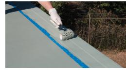
Re-coat based on manufacturer's recommendations regarding proper drying time.
