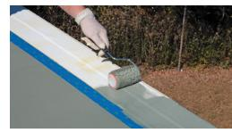
Once primer is dry to the touch, apply the first coat of paint.
