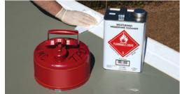
Clean the surface to be painted using Carlisle's Weathered Membrane Cleaner and allow to dry thoroughly.
