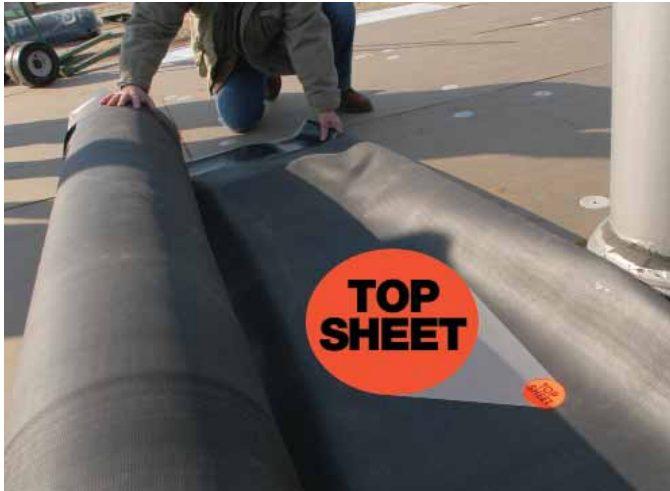
Locate the orange TOP SHEET sticker on 2-packs to ensure proper roll-out.
