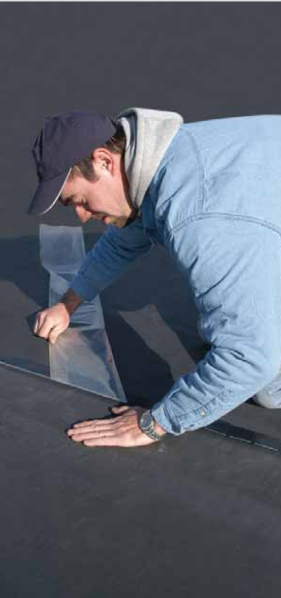
Seams completed with Versico's QAT Seam Technology go together smoothly, resulting in fewer wrinkles.
