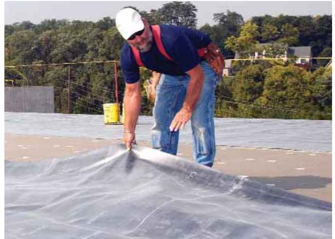
VersiGard EPDM with Quick-Applied Tape formats for wide-width sheeting includes a single-fold sheet.
