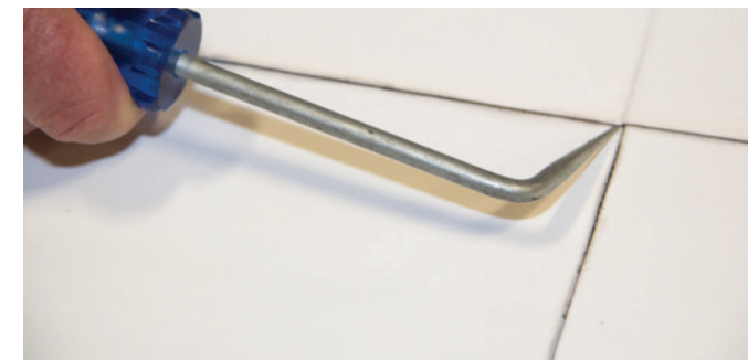
INCORRECT. HEEL DRAG CAN CAUSE DAMAGE TO MEMBRANE.
