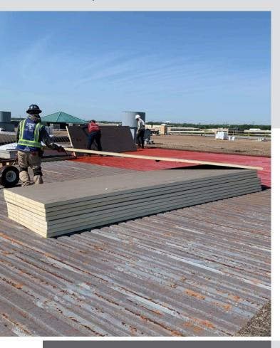
Versico Roofing Systems' introduction of 12' VersiCore flat polyiso brings labor savings and efficiency to get more done in less time. With fewer panels to load onto the roof and less time spent positioning, 12' VersiCore is the most efficient insulation option for large-scale jobs.
