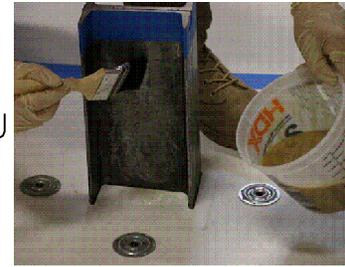
PRIME I-BEAM AND METAL PLATES. ENSURE AMBIENT AIR TEMPERATURE IS 40° & RISING. ALLOW PRIMER TO CURE UNTIL TACK-FREE.
