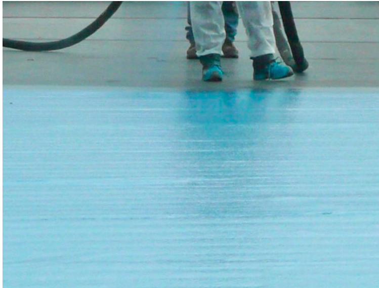
Fig 1. Full Spray Application
