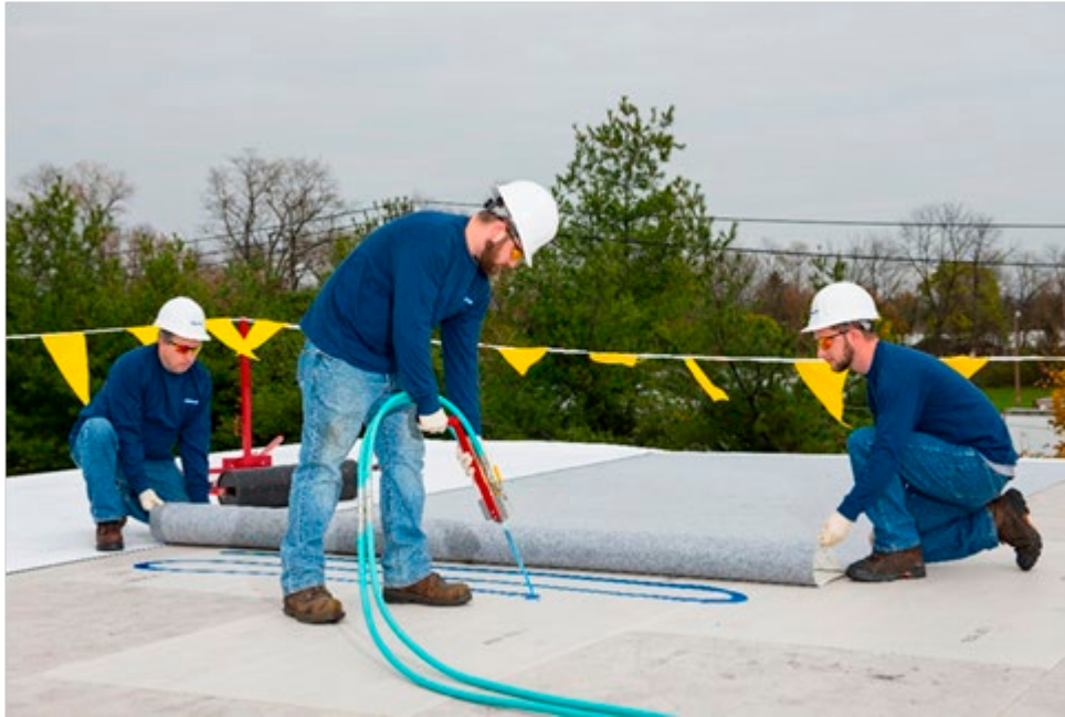
Fig 2. Bead Application
