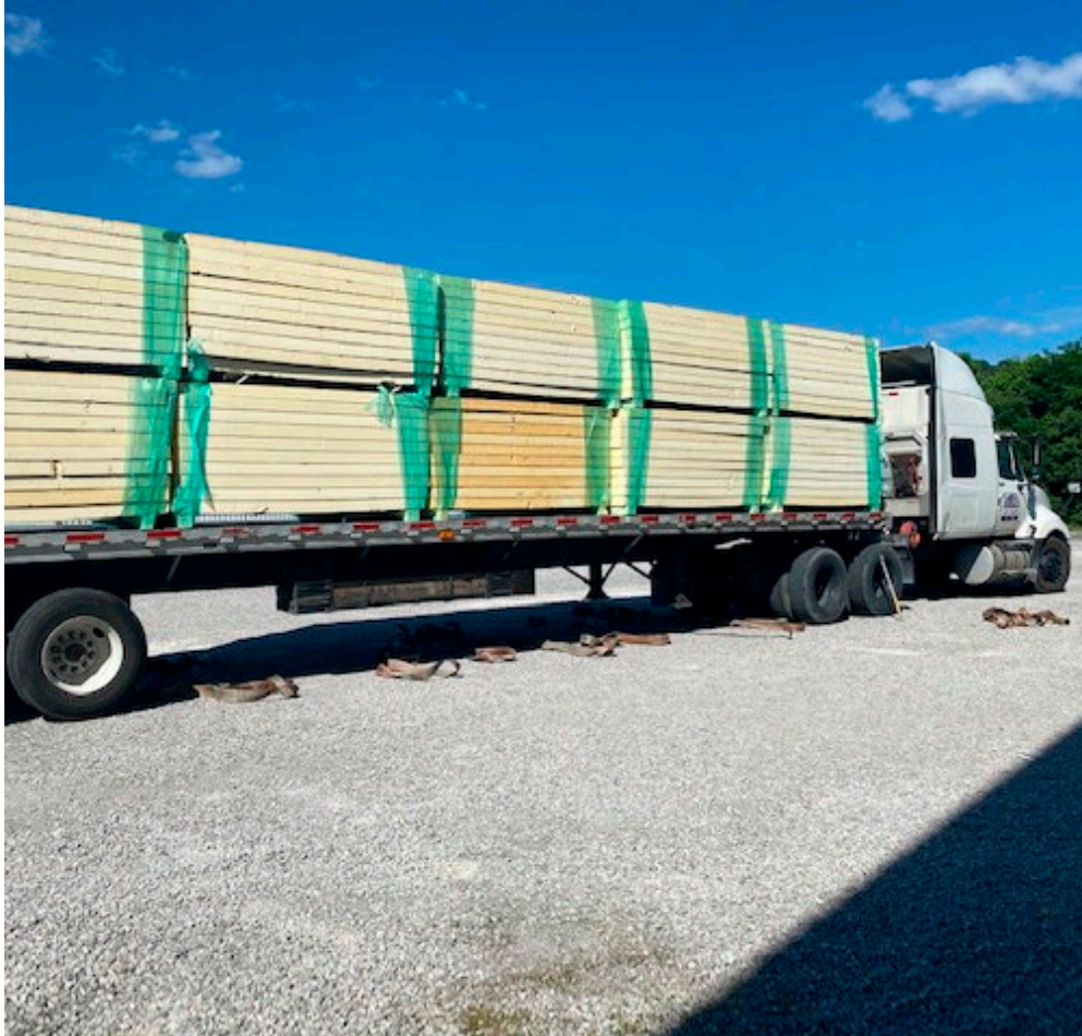
Foam board insulation is removed, stacked and loaded on a trailer.
