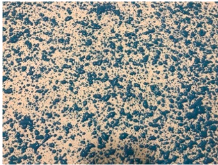
Fig 3. Correct Coverage – Splatter Application
