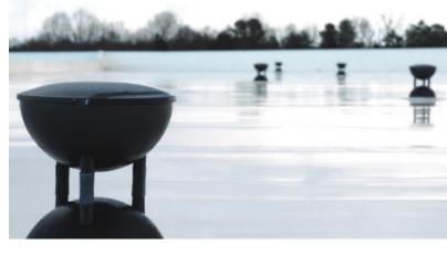
with any loose-laid system. The VacuSeal System has achieved uplift testing at Underwriters Laboratories, see TGIK.R25921 for results. If the designer or building owner is looking to meet certain uplift criteria based on FM designations, we can provide calculated uplift pressures of our system to relate to their requirements. If it is FM-insured it is more of a challenge; we have been accepted on FM-insured projects, but it is burdensome.
