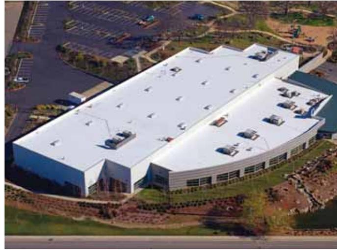
KEE HP has a proven history of performance. It has an improved chemical resistance and higher molecular weight compared to standard KEE. It has improved aesthetics, better thermal performance, a wider window of weldability, and improved cold temperature flexibility, making it an ideal roofing membrane for virtually any condition.
