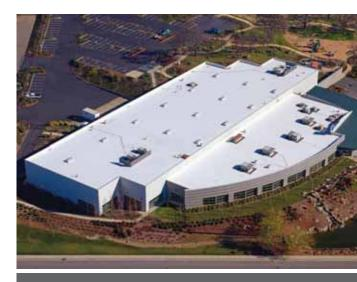
KEE HP has a proven history of performance. It has an improved chemical resistance and molecular compared standard improved aesthetics, performance, a wider window of weldability, and improved cold temperature flexibility, making it an ideal roofing membrane for virtually any condition.
