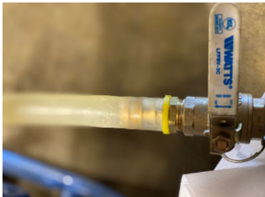
Fluid Valve (closed position)
