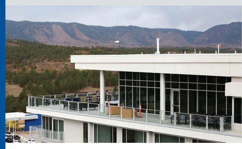
The roof over the hotel has hundreds of penetrations that had to be carefully flashed, including internal and overflow drains, vent stacks, and a recessed mechanical well. In addition, there were 120 davits installed across the center of the roof to support window washing equipment. For the smaller pipe penetrations and davits, the DCG team installed pre-molded TPO pipe boots welded to the deck and sealed at the top with Water Cut-Off Mastic and a stainless-steel pipe clamp.
