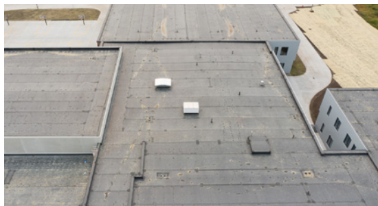
Carlisle's FleeceBACK RapidLock (RL) EPDM remains intact after derecho storm hit Marion, IA.
