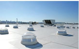
FleeceBACK membranes have a tried and true record of exceptional puncture resistance, and feature up to 75% fewer seams than modified bitumen roofing systems – providing applicators with significant labor savings.
