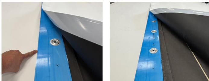
**Step 4:** Remove the outside section of the blue split SeamShield film as well as the gray film on the underside of the sheet, exposing a clean, weldable area. These can be pulled individually or at the same time. Wait until you are ready to weld to do this step to ensure the seam stays clean.
