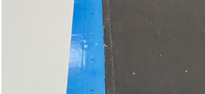
**Step 2:** Line the adjoining sheet up with the top of the X's, ensuring at least a 2" overlap of the two TPO sheets.
